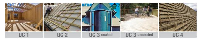
\* In accordance with EN 335: 2013 Use Class 3 COATED can also be referred to as 3.1 and Use Class 3 UNCOATED as 3.2.
